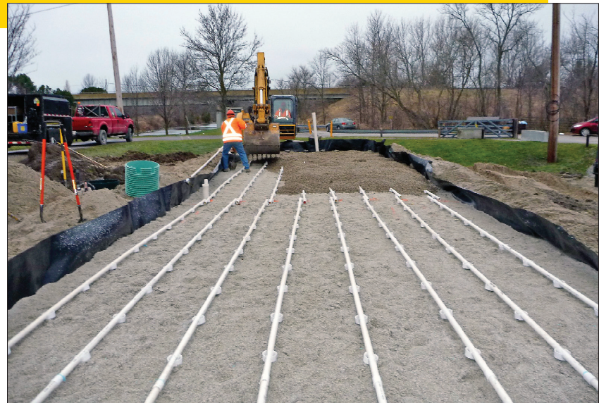
Kirk Hastings adds the final layer of aggregate above the distribution piping while his assistant rakes and levels it. (Photos courtesy of Centre for Sustainable Watersheds)
