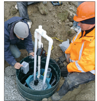
Étienne Bordeleau (left) and Kirk Hastings verify the placement of the Biotube pump vault and final location of the float level alarms.
