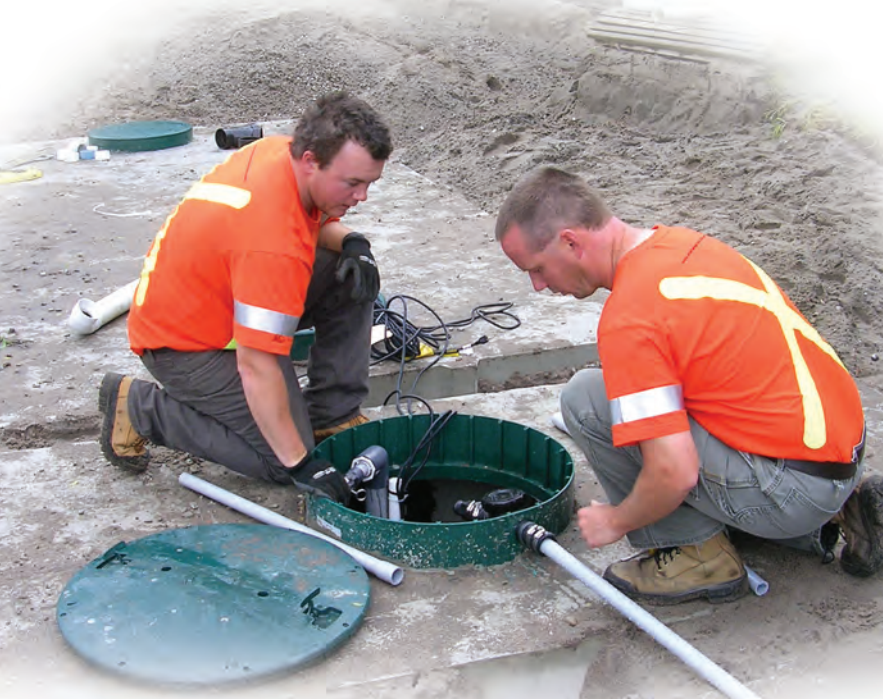
Upper photo: Mac McGill (left) installs a time-dosed pump system as Kirk Hastings assists. At right, a 3-inch polyethylene sewer line is installed behind a high-pressure horizontal drilling head.
