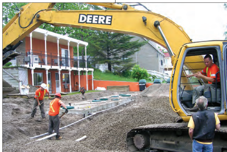
Al Lalonde (back left) and Mac McGill construct a force main, while Kirk Hastings (in excavator) consults with property owner.
