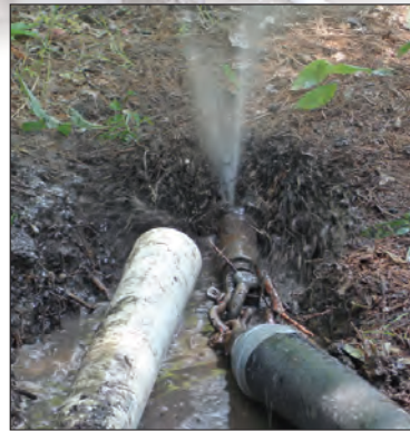
Upper photo: Mac McGill (left) installs a time-dosed pump system as Kirk Hastings assists. At right, a 3-inch polyethylene sewer line is installed behind a high-pressure horizontal drilling head.
