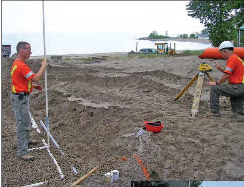
**Above, Kirk Hastings recalibrates the drainfield's elevation, while Allan Lalonde adjusts the slope laser. At right, spray foam insulation was applied 3 inches thick over the concrete components to prevent the microbes from freezing in winter.**
