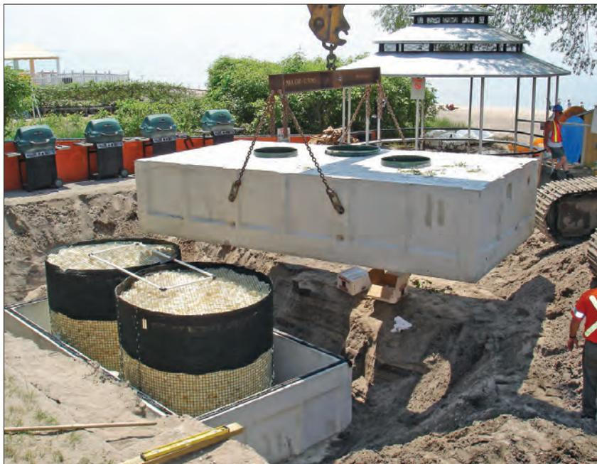
A crane operator places the top of the biofilter container tank over the foam media and distribution system.
